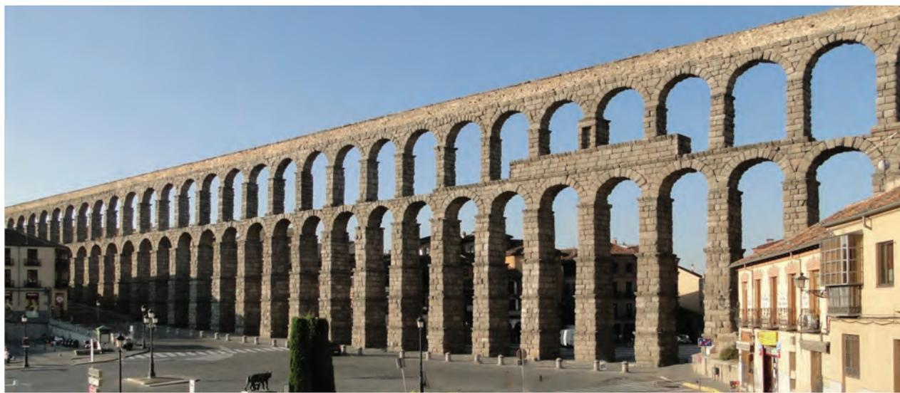
*The Roman aqueduct in Segovia, Spain, stands as one of the most well-preserved and astounding engineering feats of the Roman Empire. Constructed around the 1st century AD, it soars to a height of 93.5 feet (28.5 meters). Remarkably, no mortar was used in its assembly. The granite blocks were meticulously cut and expertly balanced, enabling the aqueduct's continuous operation in delivering water to the city until the 19th century.*
