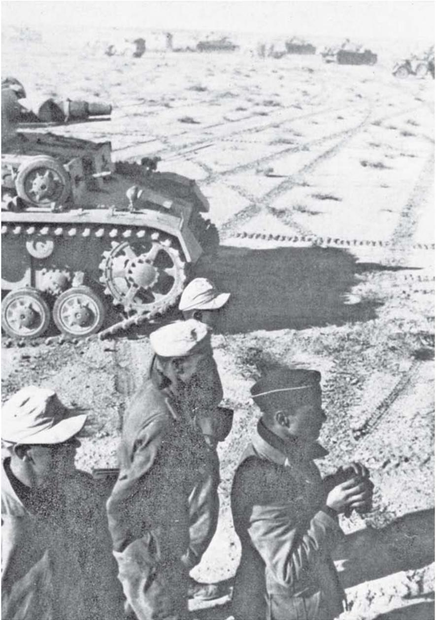
*Panzers ready to advance. A Panzer IV Ausf. E with its short 75mm main gun and bolted-on supplemental armor is in the background.*
