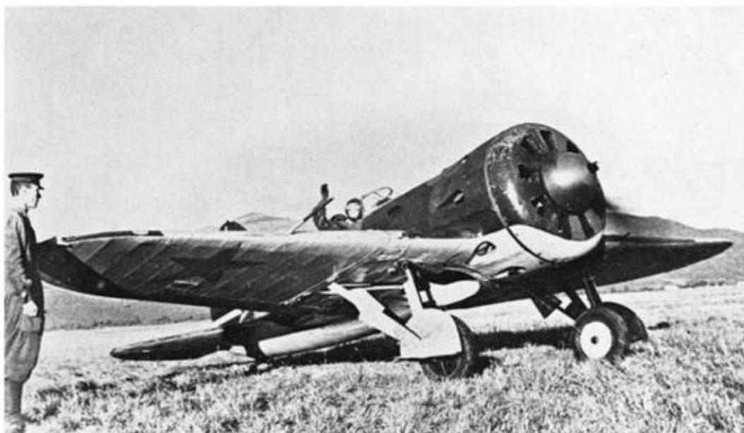
The world’s first cantilever-winged monoplane fighter with retractable landing gear, Polikarpov’s I-16 formed the backbone of the Soviet Air Force at the time Hitler’s forces invaded Russia. Nicknamed Ishak (“Donkey”) by its own pilots for the I-16’s unpleasant, even potentially life-threatening flight characteristics, it was decimated in combat. (Courtesy Art-Tech)
