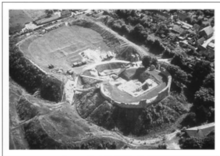
**Figure 13.4** Castle Acre, Norfolk, a castle with inner and outer bailey connected by a bridge. The keep of the 1140/50s was converted from a weakly defended house dating from the eleventh century; refortification included heightening the perimeter bank and adding a curtain wall.
