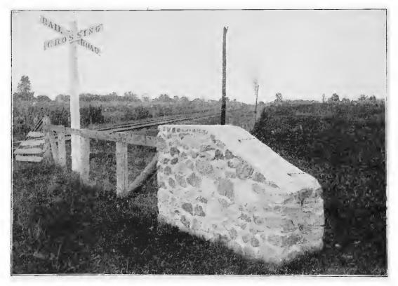
FIG. 251-STONE ANCHOR-WALLS FOR FENCE.
