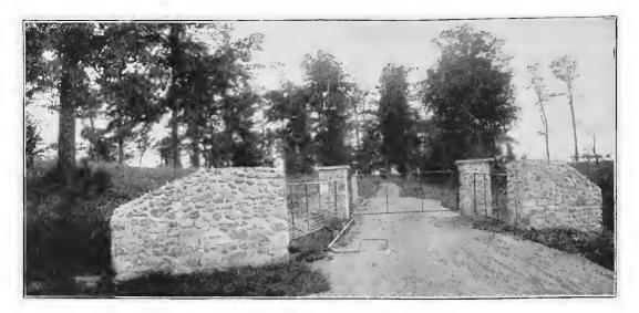
FIG. 250-STONE ANCHOR-WALLS FOR FENCE.
